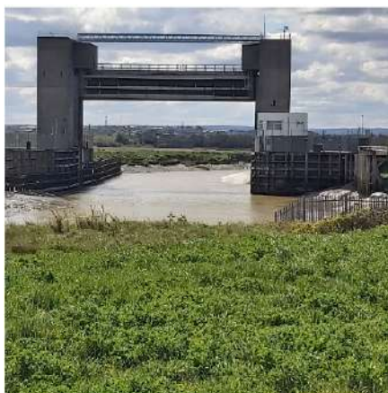
Dartford Creek Flood Barrier
